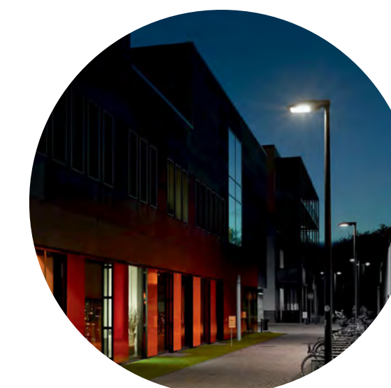
16 Post mounted lighting for parking and driveway lane
